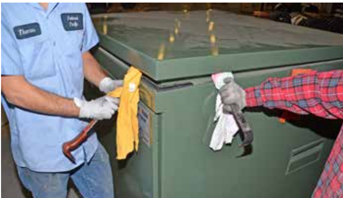
Figure 4. Using pry bars to "break loose" the roof gasket attachment. Protective measures, such as wrapping the pry-bars with cloth as shown should be used to protect enclosure finish( paint).
