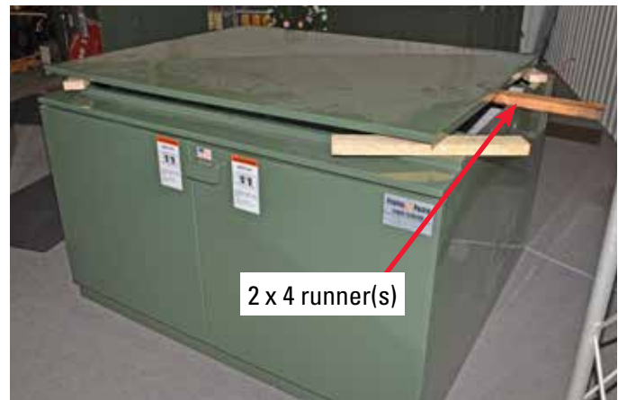
Figure 6b. Cross-piece runner board(s) is (are) installed to aid in removal of the roof and are normally installed in the direction the roof will be moved.
