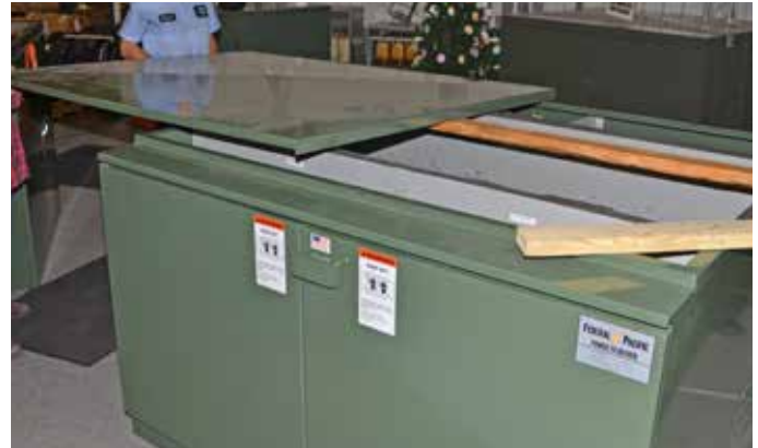
Figure 7. PSE roof moved to side to allow work on switchgear.
