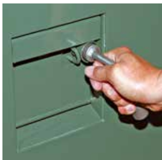
Figure 10. Door handle cover is secured closed by a penta-head (or hex-head) bolt. Turn socket counter-clockwise to loosen bolt.
