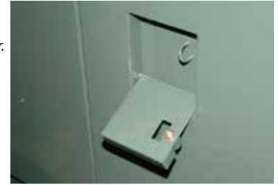
Figure 11. With penta-head bolt fully loosened, handle can be pivoted down to unlatch the door.
