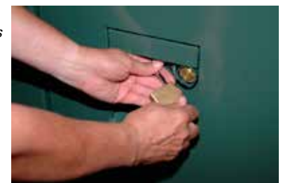
Figure 13. Padlock cannot be inserted until penta-head bolt is fully tightened.
