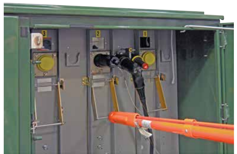
Figure 25. Shotgun-clamp stick secured to interlock lever.
