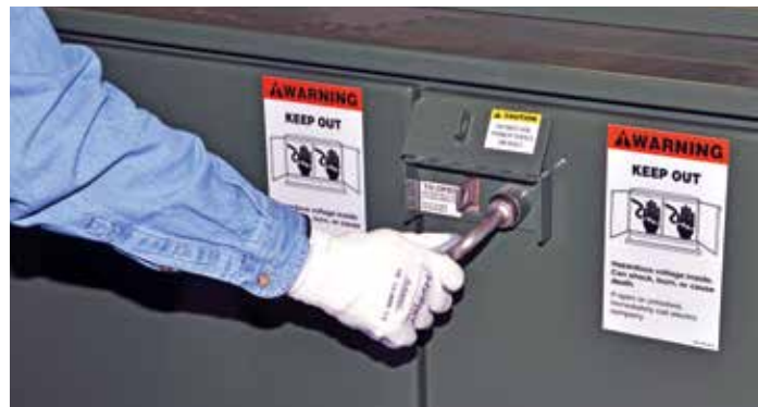
Figure 4. Use a manual wrench with pentahead or hexhead socket as applicable. As explained on the caution label, DO NOT USE POWER TOOLS . Rotate the security bolt clockwise or counter-clockwise to release three-point latch and charge for subsequent door closing. Do not use power tools to operate the security bolt.
