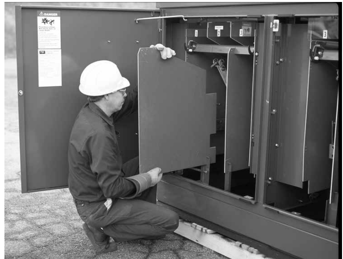
Figure 8. Switch-side removable barriers facilitate cable installation and termination. Lift up and pull out to remove barriers.
