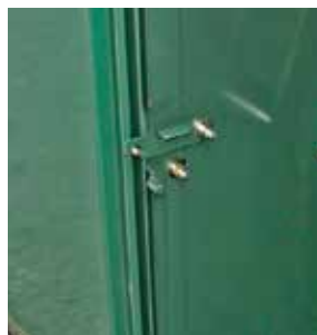
Figure 2b. Release passive door by simultaneously pushing on it and raising the latch bracket.
