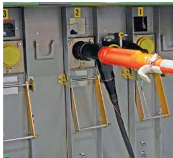
Figure 21. Shotgun clamp stick secured to elbow for removal/connection.
