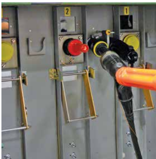
Figure 23. Shotgun clamp stick secured to elbow with elbow moved to feed through stand-off bushing on parking stand.
