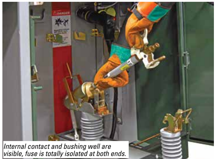
Figure 33. Alternate method using insulating-gloved hand, if user's standard operating procedures permit, to remove fuse from fuse mounting.
