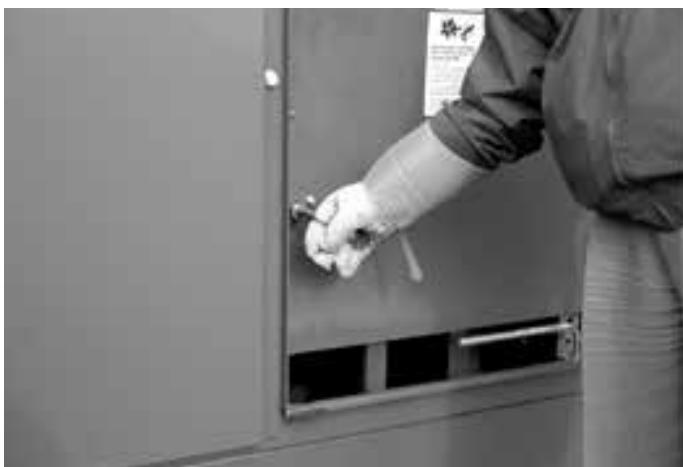
Figure 9. Disengage barrier security bolt using pentahead socket.
