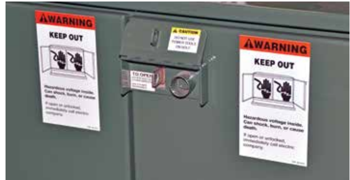
Figure 3. Raise cover to access security bolt. Review and understand the “CAUTION” label on the underside of the cover.
