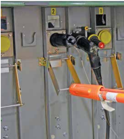
Figure 26. Interlock lever being raised to unlocked position (or lowered to locked position).
