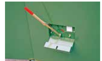
Figure 15. Place handle socket on switch-operating shaft. Rotate handle in direction as indicated.
