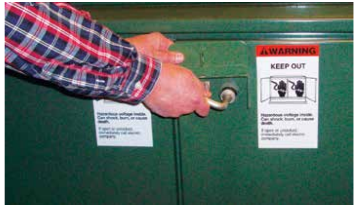
Figure 33. Raise cover to access security bolt. DO NOT USE POWER TOOLS ON THIS BOLT.
