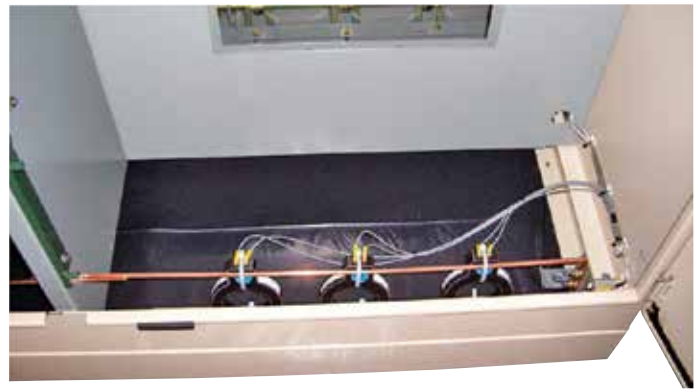
Figure 17.d. Current-sensing transformers for the Self-Powered Relay are shown tie-wrapped to the ground bar as arranged for shipment and are to be secured to the cable using heavy-duty tie wraps. Current sensors must be installed below the terminator. The concentric-neutral wires must pass back through the current sensor before being taken to ground as described on page 11.
