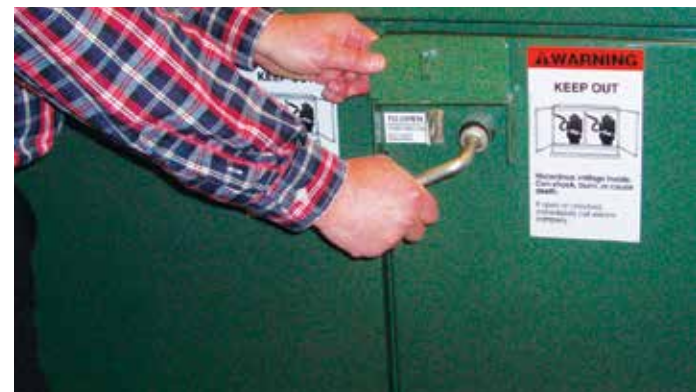
Figure 34. Wrench with pentahead socket or hexhead socket as applicable. Rotate bolt clockwise or counter-clockwise to release three-point latch and charge for subsequent door closing. DO NOT USE POWER TOOLS ON THIS BOLT.
