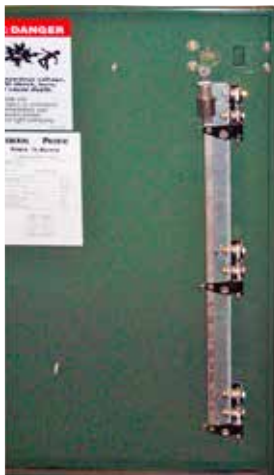
Figure 32a. Auto-latch mechanism with 3-point latching on door closure.
