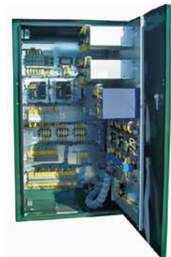
Figure 18b. Shown above is a view of a typical low-voltage compartment used when the SEL-501 relay, which is mounted on a hinged-bolted panel, is selected as the overcurrent relay to use in the protection scheme. In this case, two relays are required as three (3) load-feeder circuits are involved. The UPS and auxiliary control components are also shown. The photo at bottom shows the interior of the low-voltage control compartment with the hinged-bolted panel swung open.
