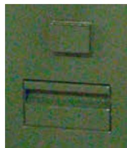
Figure 11. Hinged padlockable cover over switch-viewing port (an alternate arrangement).
