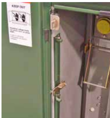
Figure 32b. Release passive door by simultaneously pushing on it and raising the latch bracket.
