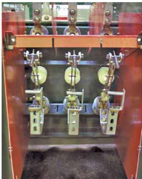
Figure 1. Switch open with interphase barriers removed. Cable connections, terminators and grounding clamps not illustrated.
