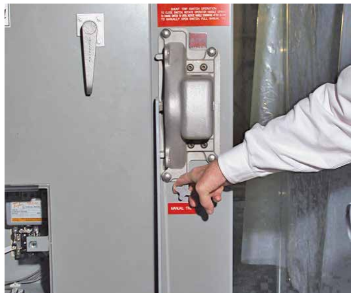
Figure 14. Manual Shunt-Trip Knob.
