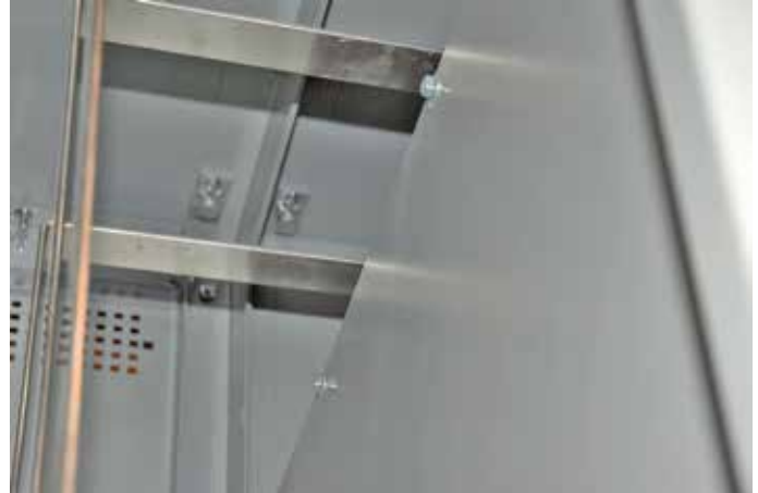
Figure 3c. Draw edges of bus openings together, if necessary.
