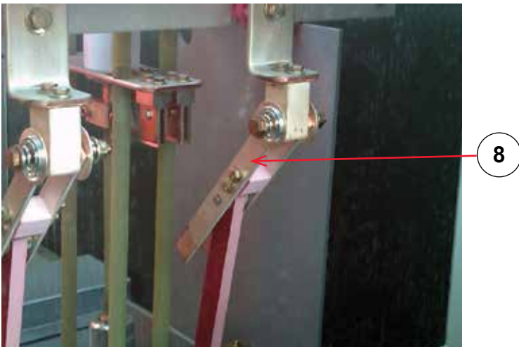
Figure 21. Integral Visible Disconnect — Disconnects Open.
