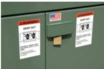
Penta-head (or optional hex-head) actuated door lockbox features stainless-steel hinged padlockable cover to block access to bolt head. Rotate bolt in either direction for opening.
