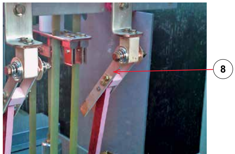
Figure 21. Integral Visible Disconnect — Disconnects Open.
