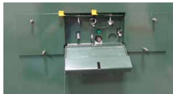
Figure 2. PROM-PM Mounting Plate secured in handle pocket.
