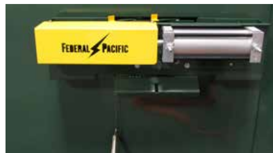
Figure 3. PROM-PM Operating Mechanism secured to mounting plate.
