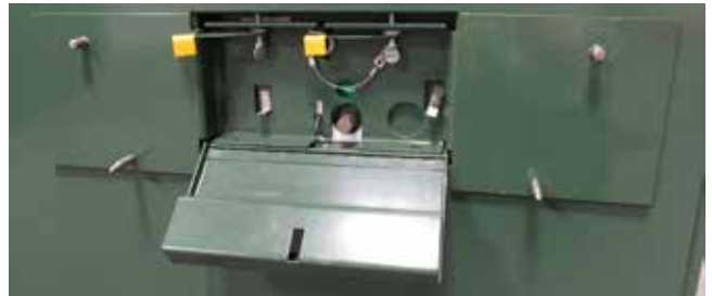
Figure 6. PROM-PM base installed in a switch operating pocket, levers to the left, and security hook installed in pocket eye hasp.
