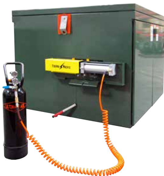
Figure 1. PROM-PM Installed on a Live-Front PSI/II Model with Tank and Hose. The same PROM-PM can also be installed on Dead-Front PSE Units.
