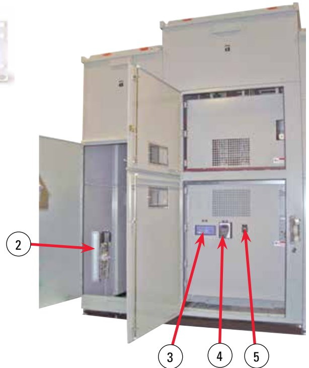
Figure 4. Bay 2 – Screens Closed
