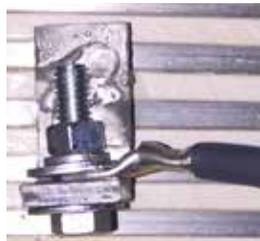
Figure 3 - Welded Terminal Pad
