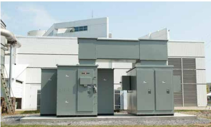
Figure 3. Automatic-transfer switchgear with Fast-Trip Transfer motor operators is pictured in the photo above. Transfer to the alternate source is achieved in approximately twenty (20) cycles.
