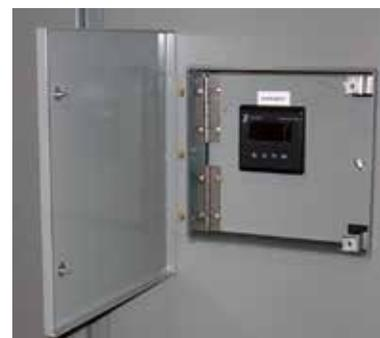
Figure 16. The digital power monitoring meter that allows real-time display of the various circuit parameters is mounted on a hinged, bolted panel in a low-voltage compartment that is isolated from high voltage.
