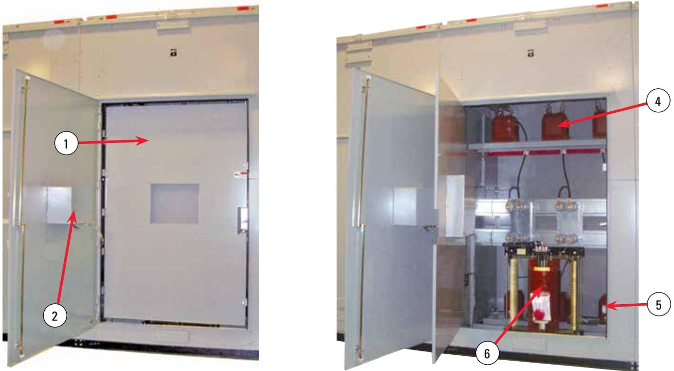
Figure 7. Bay 4 — The Customer Metering Bay with an Advanced Metering Relay is pictured above and in inset below.
