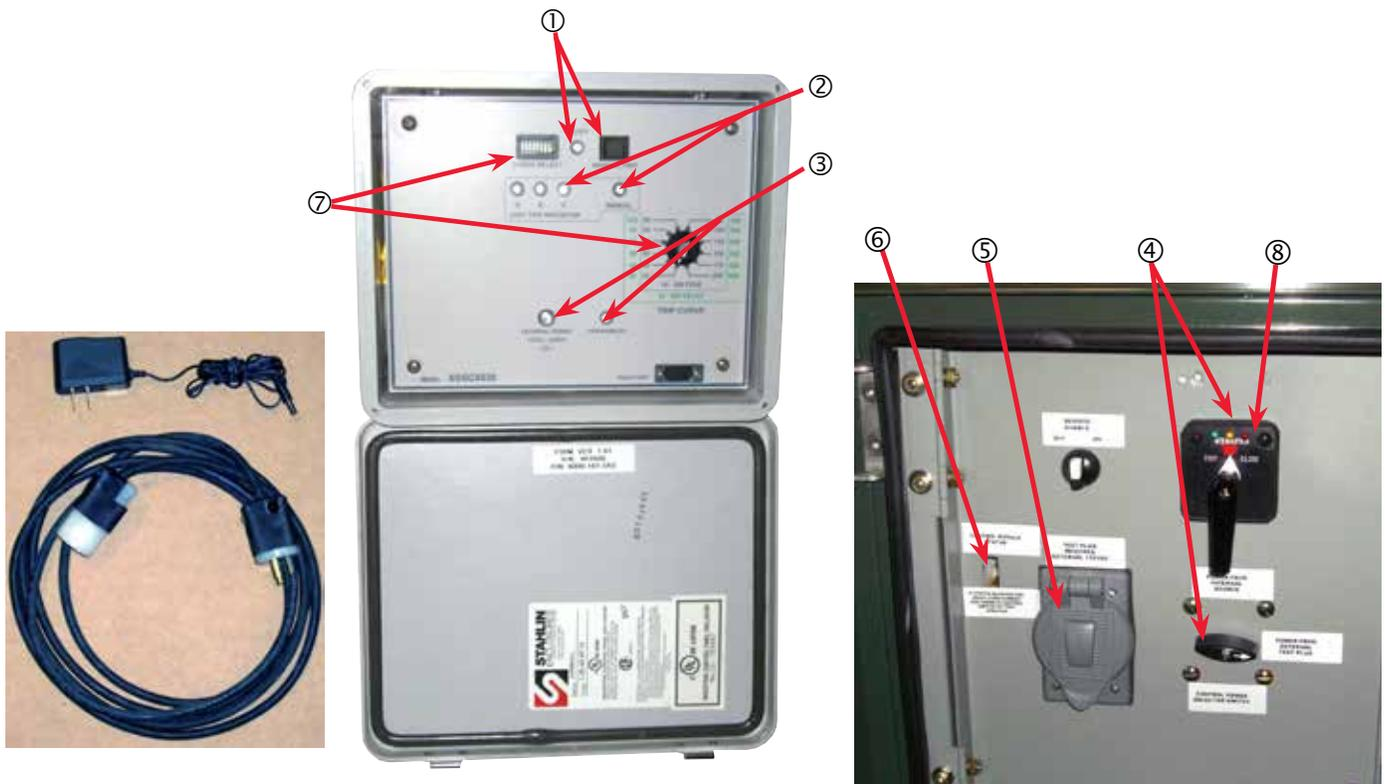
Figure 3. Faceplate of Self-Powered Relay is at center and Control Panel is at right and both are inside the Low-Voltage Compartment. A ten-foot extension cord (at bottom in left photo) is provided for connection of an external 120vac control-power source and a 120 vac/12v dc power cord (at top in left photo) is provided for control power to the self-powered relay.
