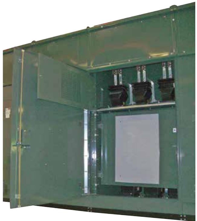
*Figure 3. Open door view of metering bay showing (at left) a hinged protective screen at top section over current transformers and a hinged- panel with a plywood section for meters and controls to be installed by the utility. The perforated screen allows viewing the CTs without opening the screen. With the screen open (in photo at right), the revenue metering, outdoor-style, current transformers are completely visible for closer inspection.*
