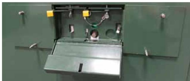
Figure 6. PROM-PM base installed in a switch operating pocket, levers to the left, and security hook installed in pocket eye hasp.
