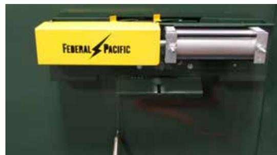
*Figure 3. PROM-PM Operating Mechanism secured to mounting plate.*
