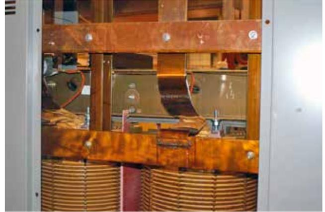
Figure 7. Brazed copper LV lead to Cu bus.
