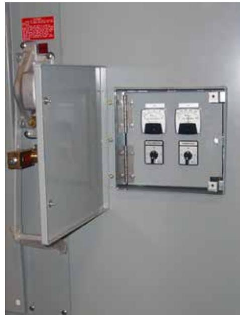
*Figure 3. Pictured above is Bay 2, which includes the incoming switch for the alternate (backup) source. Insets show (at top) screen over the switch that is encountered when the enclosure door is opened and (at bottom) the analog voltmeter and ammeter with selector switch, allowing a real-time verification of the condition of the incoming power source. Bay 1, which includes the incoming switch for the preferred (normal) source is similar.*
