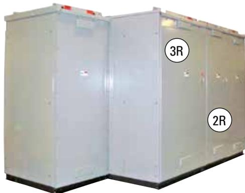
*Figure 1. This six-bay lineup of 25kV Manual Metal-Enclosed Switchgear is arranged in a back-to-back configuration with four (4) bays in the front (in the two top photos taken from the left side and from the right side) and two (2) bus-transition bays in the rear (in the photo at left). The configuration allows the medium-voltage distribution switchgear with a vacuum circuit breaker to better match the available space at the installation site.*
