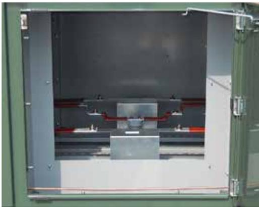
*Figure 7. This is a close-up view of the interior of Compartment 5 through the panel opening. The steel support plates visible in the bus at the bottom of the switchgear metering unit are temporary bus supports which will be removed and replaced by the bar-type CTs, to be installed by the customer.*
