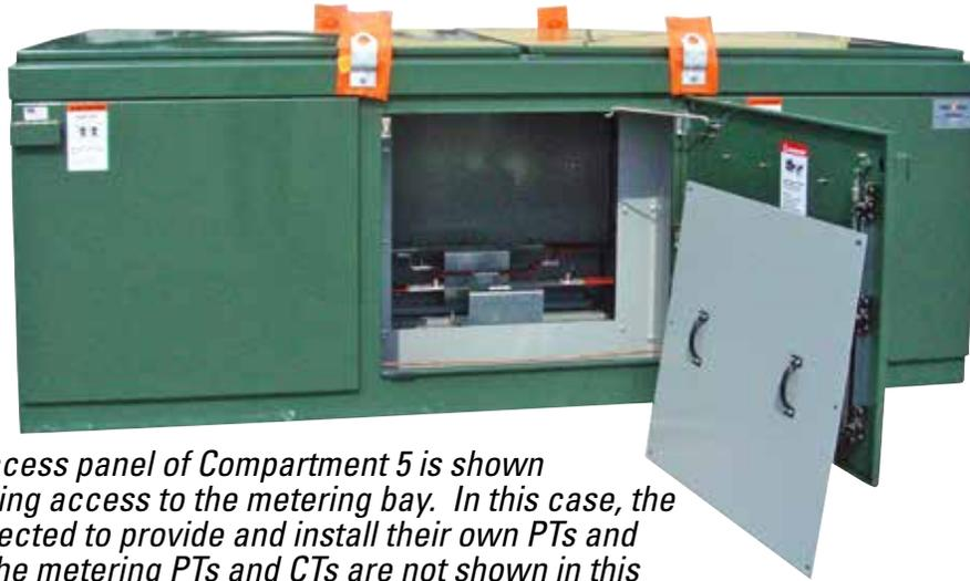
*Figure 6. The access panel of Compartment 5 is shown removed, providing access to the metering bay. In this case, the customer has elected to provide and install their own PTs and CTs, therefore, the metering PTs and CTs are not shown in this illustration.*
