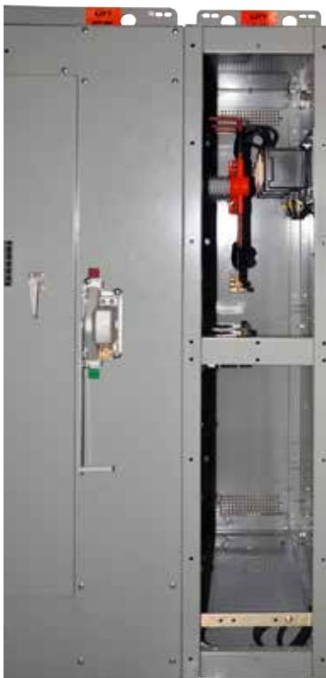
Figure 6. Three (3) 4.16kV voltage transformers are furnished in each incoming termination compartment (Bay 1 and Bay 19). Each set of VTs provides voltage sensing input to the power monitoring unit in the associated main incoming fused switches, which are in Bay 2 and Bay 18. The voltage input combined with the current input allows the meter to produce all of the associated measurements: phase voltage, line-to-line voltage, average voltage, power factor, kW, kWh, etc.
