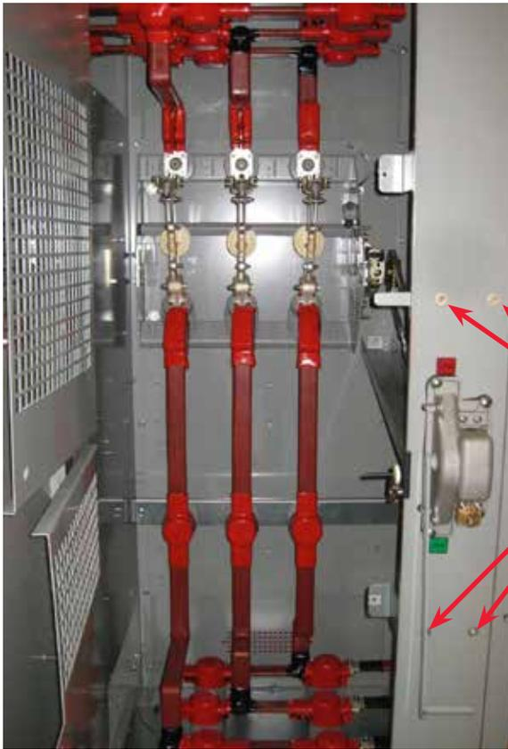
*Blind-Tapped Threaded Inserts Above and Below Switch-Operating Handles are Mounting Provisions for the Federal Pacific Portable Remote Operating Mechanism (PROM), Which is Available as a Separately Purchased Accessory, to Allow Switches to be Operated from an Adjacent Location and Thereby Mitigate the Effects of any Potential Arc-Flash Hazard (see Page 8).*
