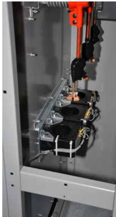
Figure 7. Three (3) 1200:5 current transformers are furnished in each incoming termination compartment (Bay 1 and Bay 19). Each set of CTs provide current sensing input to the power monitoring unit in the associated main incoming fused switch, which are in Bay 2 and in Bay 18. The current input combined with the voltage input allows the meter to produce all of the associated measurements: phase current, average current, kW, kWh, etc.
