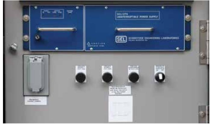
*Figure 7. The Federal Pacific automatic-transfer scheme includes a UPS (at top in photo), test pushbuttons to simulate loss of source voltage and over-current lockout to allow verification of the functionality of the transfer scheme, and a duplex outlet for connection of a laptop computer. Also see Figure 6.*
