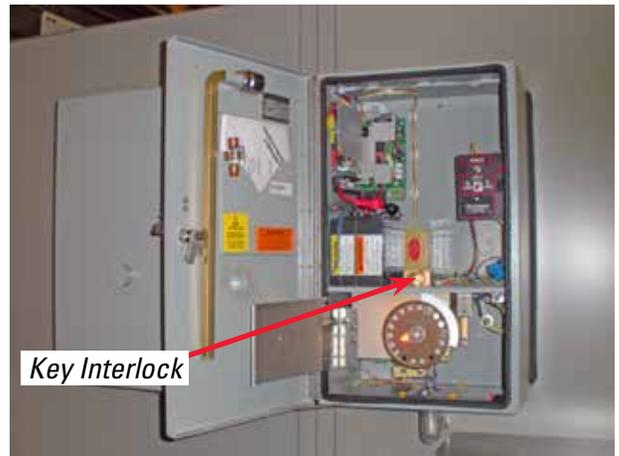
*Figure 5. The Fast-Trip Motor Operator is illustrated above with the interlocked cover over the motor shown closed in the top photo above and with the cover open in the bottom photo above. As the motor rotates at high speed, if the cover is open motor operation is suspended. A separate key interlock (see arrow in photo) can be provided to block operation of the motor operator for other specific requirements, such as requiring that all switches be open before allowing access to fuses.*
