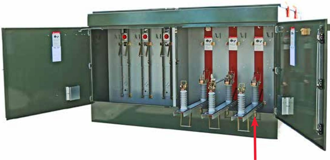
Figure 6. Fuse panels are shown open in one fuse compartment, revealing the typical shutter barrier that closes over the opening to maintain isolation of the interior high-voltage compartment. Fuse assembly is shown installed in center phase. Note that fuse panels are locked down using the locking bracket that secures the fuse panel to the door-opening flange (at arrow).
