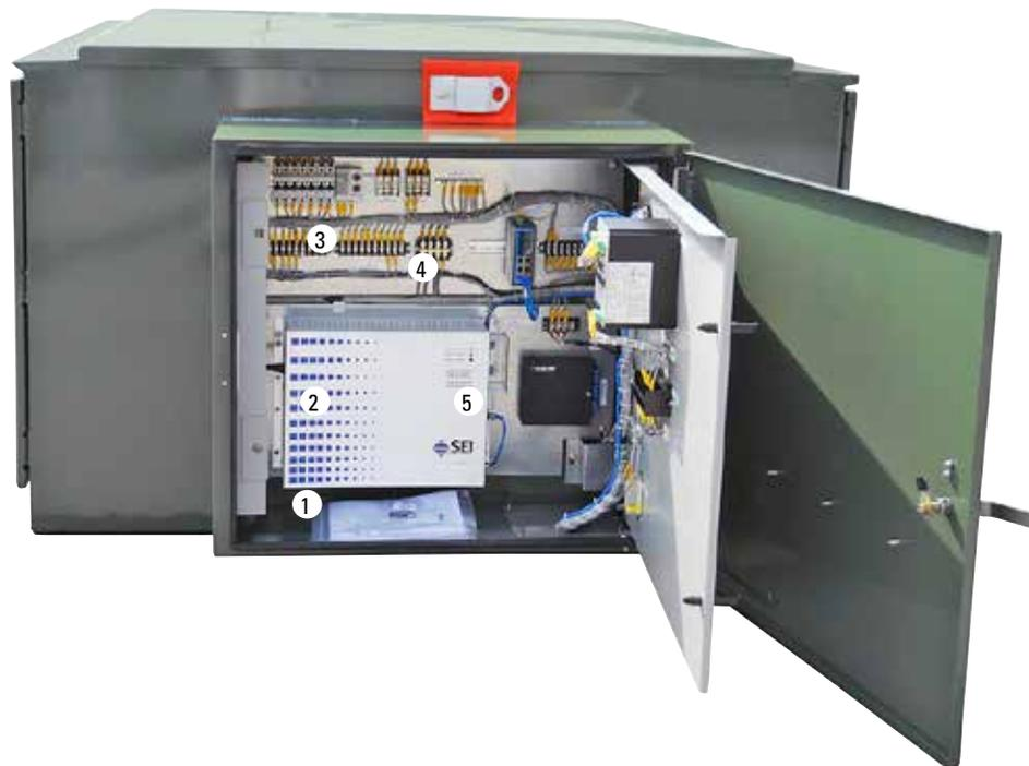
*Figure 6. Opening the hinged panel provides access to the remaining low-voltage components. Included are (1) the instructions and drawings on the bottom plate; (2) an SEI UPS Power Supply; (3) secondary circuit breakers, thermostat and heater (not visible); (4) an Ethernet switch; (5) a Black Box patch panel, and all the associated terminal blocks.*
