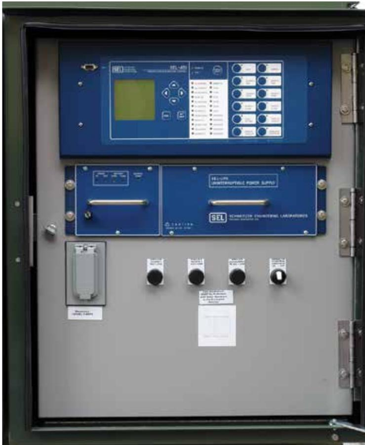
Figure 1. View of typical low-voltage control cabinet (above) that includes the automatic-transfer control relay and associated components.
