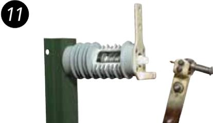
The process from the instant the switch blade starts to move until circuit interruption is achieved takes only 5 cycles.
