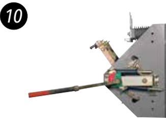
Switch Open. The switch blade has moved to the fully open position.
