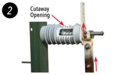
Quick-make quick-break mechanism on switch is charged using manual handle and discharges to open switch.
