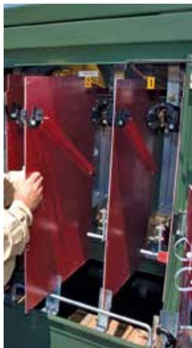
*Fuse compartments (at right) shown with dual-purpose barriers in temporary storage position on door, in alternate slide-in position on center phase of left compartment (barriers should **not** be left in alternate position for more than one week and in normal hanging position on right compartment).*
