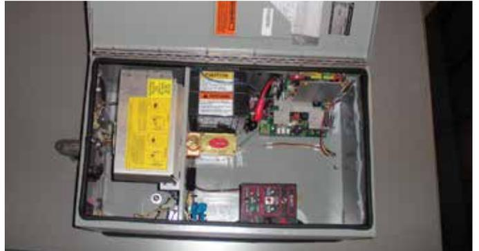
Figure 3. Fast-Trip Style Type PM Motor Operator has a larger, high-speed motor and space to accommodate an array of communications and control components similar to the Standard-Style Motor Operator. Cover (with yellow label) over motor is interlocked so that when the cover is open, motor operation is blocked to prevent exposure to fast moving parts.
