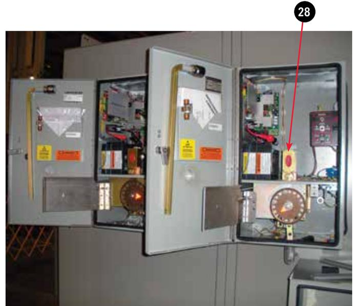
Figure 8. Open door view of Fast-Trip Style Type PM Motor Operator showing motor and decoupler lever.
