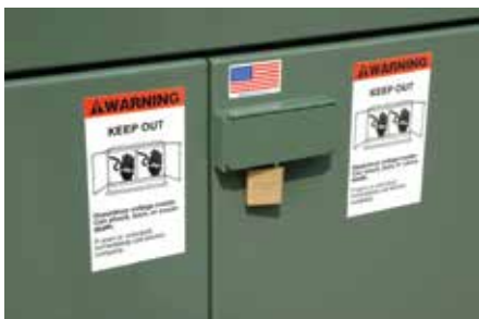
Switch-Handle Lockbox of stainless steel and is padlockable
