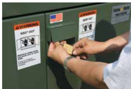
Switch-Handle Operation - handle unfolds and clip slides over joint to fix handle in extended position
