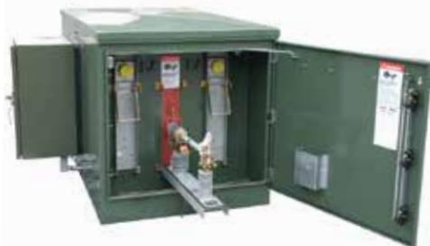
*Fuse compartment of dead-front SCADA Controlled unit is pictured above.*
