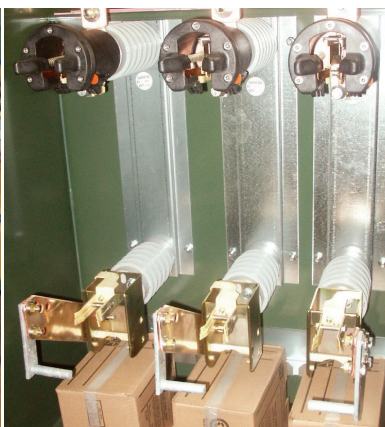
Figure 2. Lubrication points on fuse mounting include three contact locations, namely, the main contact, forward contact and fuse hinge contacts.
